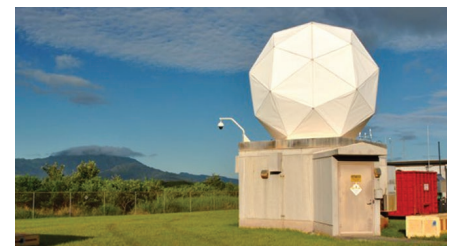
Nearby pineapple fields and other agricultural lands (top), surround and protect the Navy's state-of-the-art Mobile User Objective System satellite dishes and narrowband tactical satellite communications system for improved ground communications for U.S. forces on the move (above).
