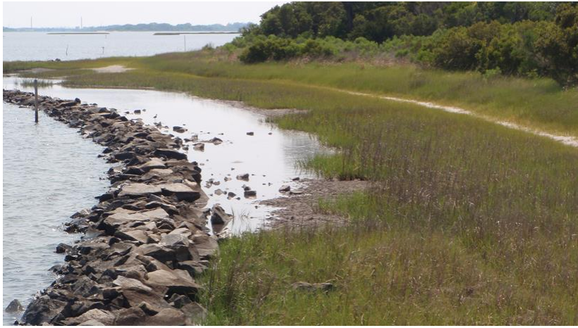
A living shoreline project on Stump Sound in Onslow County. Photo credits: North Carolina Coastal Federation.
